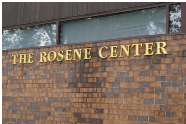
Pictured above is the "Rosene Center" lettering on the North side of the building. Similar lettering is on the South side.
